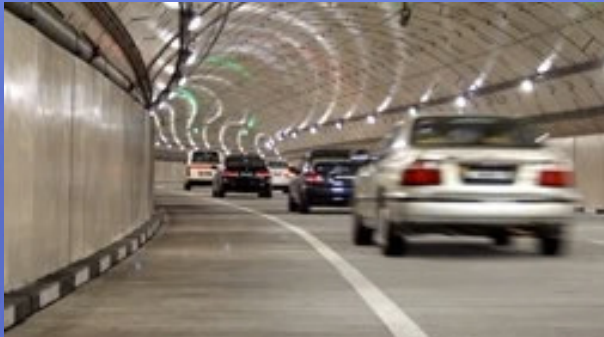
Stormwater Management And Road Tunnel (Smart), Malaysia
